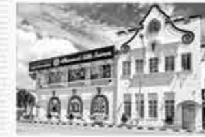
The Old Chartered Bank Building 1874
