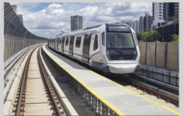
Phileo Damansara MRT Station
